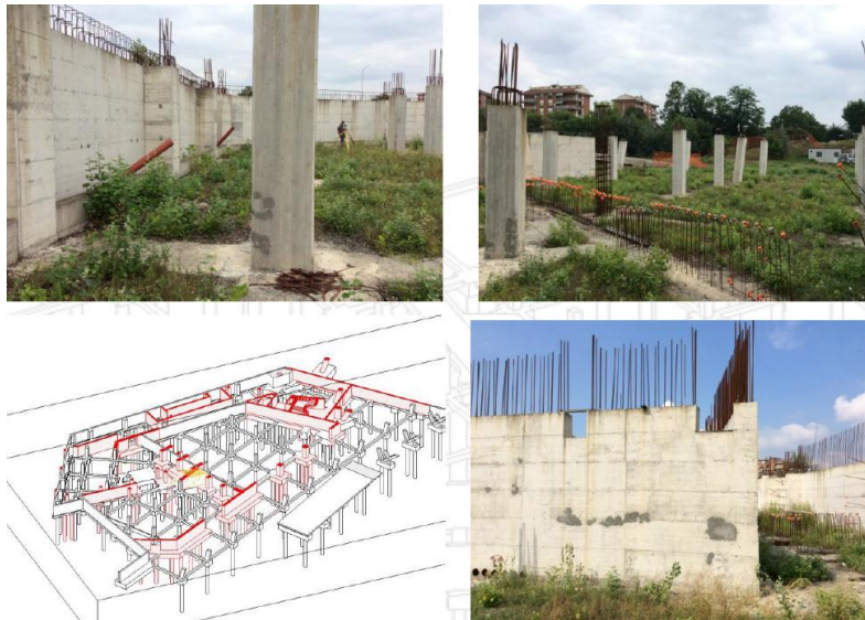
Fig. 2. Existing foundation elements and underground concrete structures.
